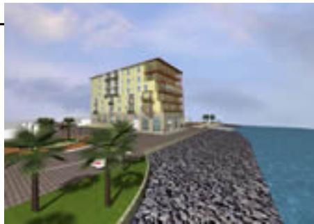
front East side
